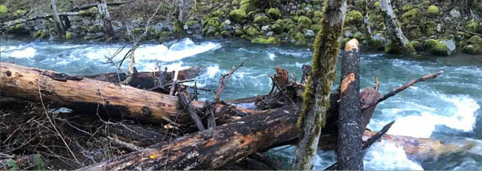
Large wood structures placed in Methodist Creek in 2017 are catching wood for future fish habitat
